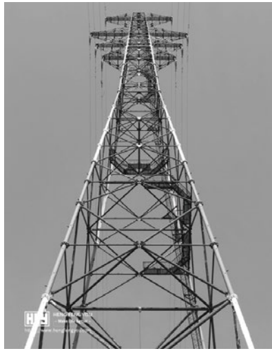
Steel Tubular Tower
