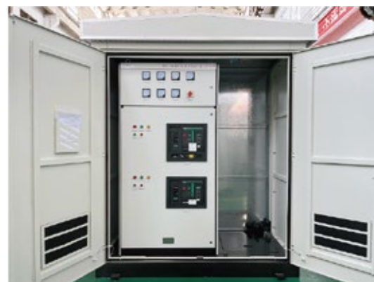
>Low voltage room-800KVA
